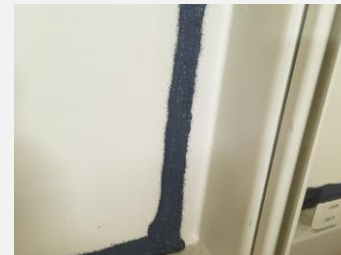
Image 2: Application of Henkel product Teroson WT 218 FR – 200. Even spray pattern, no overspray, non-sag material. Source: Henkel
